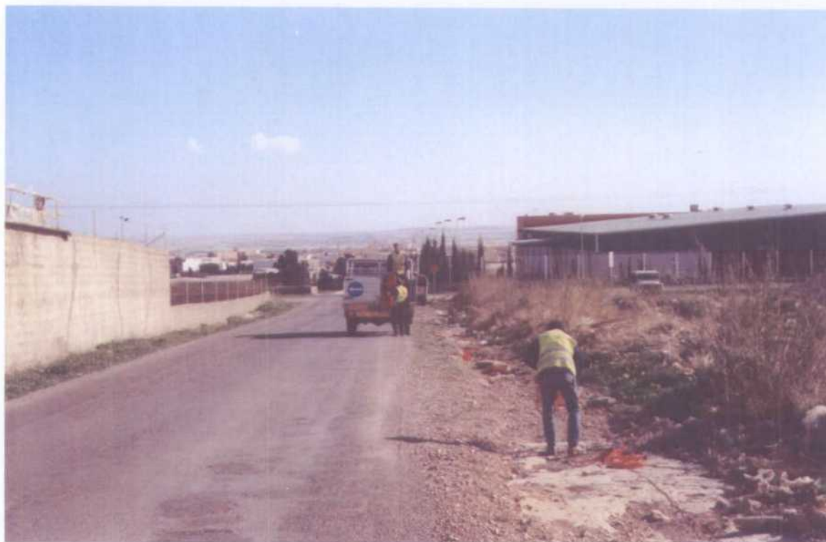
Front crew working along road and police assistance
